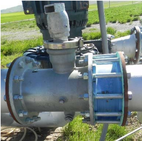
Wafer Check Valves and Spools
