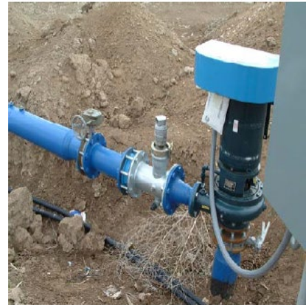
Wafer Check Valves and Spools
