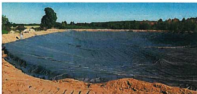
Figure 10D-6 Agricultural waste storage impoundment lined with a geomembrane ( Photo credit NRCS )
