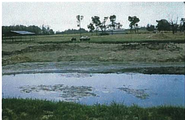
Figure 10D-24 Failure of compacted liner from uplift forces below clay blanket (Photo credits NRCS, TX)
