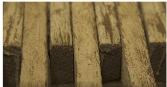
Example: wooden table with a rough, uneven surface.
